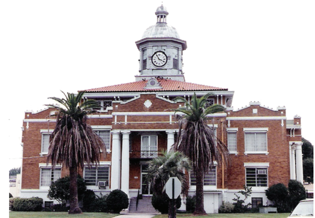
Citrus County Historic Courthouse
